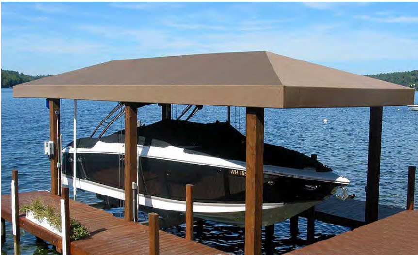
Examples of Acceptable Dock Shade Structures with low-slope hipped fabric roof in natural and earthy colors
