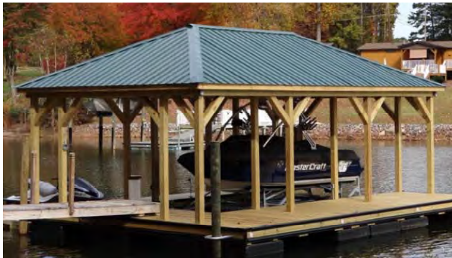
Examples of acceptable and preferred Dock Shade Structures with: open sides; low-slope hipped metal roofs; and natural and earthy colors.
