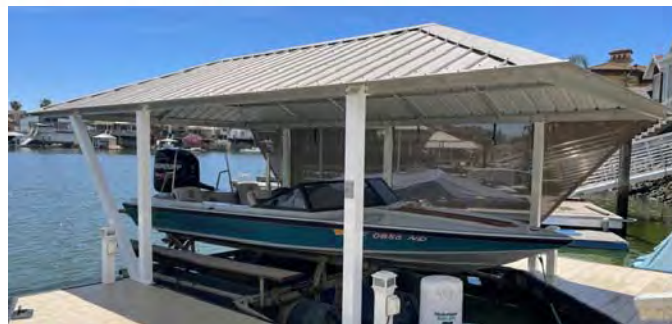
Example of a Sunscreen at Dock Shade Structure
